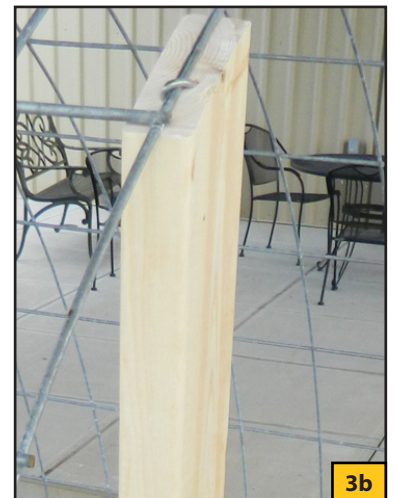
Attach uprights to the hoop with fence staples.
